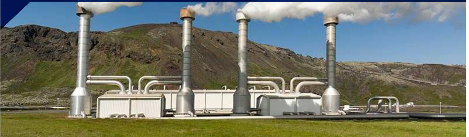
In high pressure and temperature geothermal wells geothermal water is extracted and flashed in a separation vessel. The flashed steam is used for power generation in a steam turbine. The remaining geothermal water still has high temperatures often in the range of 160°C. This water has still a high potential for power generation in a ORC where a working fluid is evaporated which is later expanded in a turbine. While evaporating the working fluid the geothermal water cools down.
